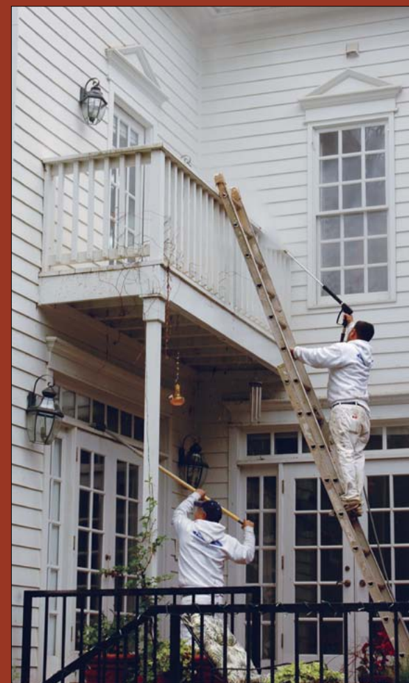
Above, bottom: A Painting Plus crew pressure washes a home in Atlanta's Buckhead neighborhood. Owner Charlie Dallavalle Jr. believes he gets better results if the crew members who paint the house also do the pressure washing.
